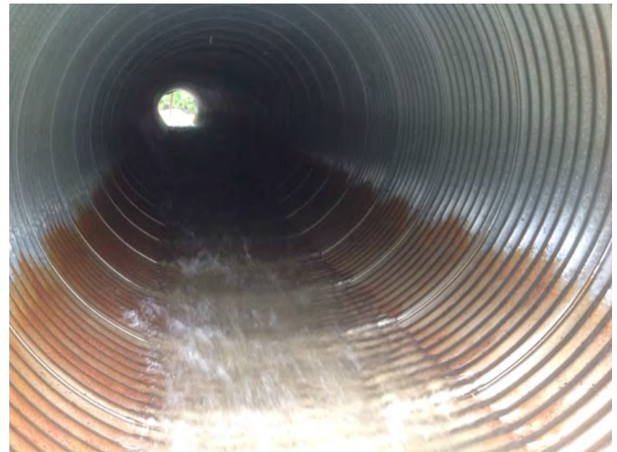
looking through culvert from outlet
